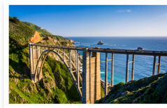
concrete road bridge
