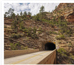
The Zion-Mount Carmel Tunnel in the USA is a tunnel through a mountain.
