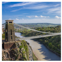
Clifton Suspension Bridge
